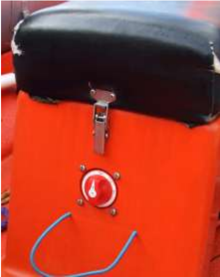
Isolator switch OFF
